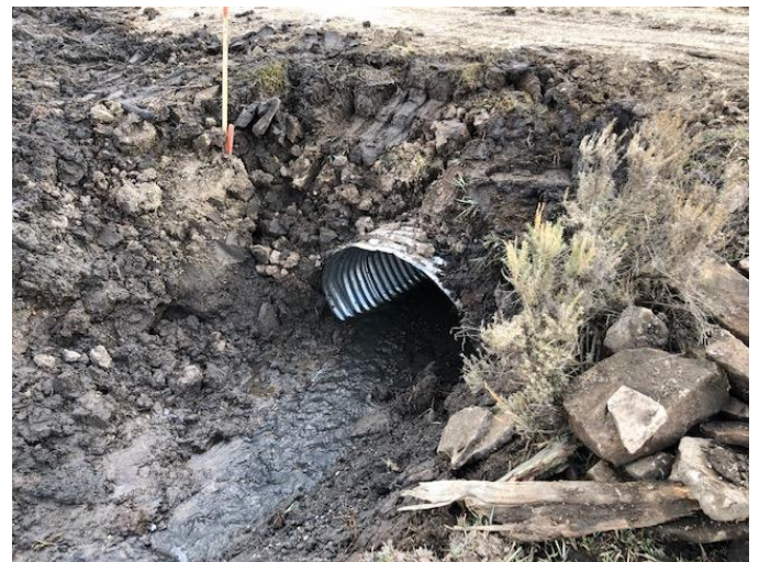
New culvert crossing installed on 1 st Creek within the Smiths Fork BLM Allotment.
